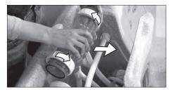
**Step 4:** Loosen the two PVC unions, pull the manifold out from in between the two water unions.
