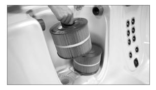
**Step 4:** Using a garden hose with a nozzle or other high-pressure device, clean cartridge(s). Work top to bottom on each pleat.
