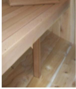
Position the bench supports under the benches as shown. Line them up with the supports on the bottom, slide them back to the wall, and screw them in place with supplied 2½" wood screws.
