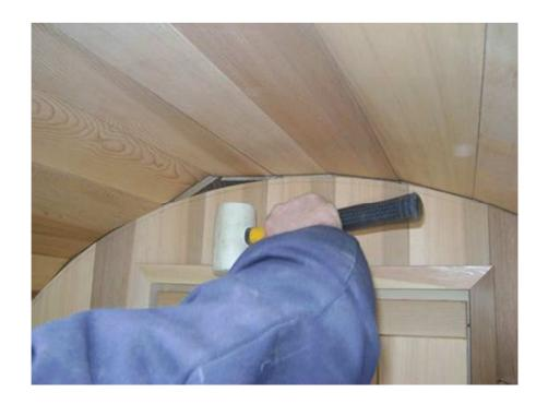
By adjusting the staves this way (bumping them up or down with a rubber mallet, as necessary) they should settle into a circular shape as pictured below.
