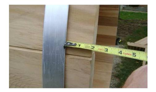
Measure 2" from the edge of the band to the end of the staves all around before tightening.
