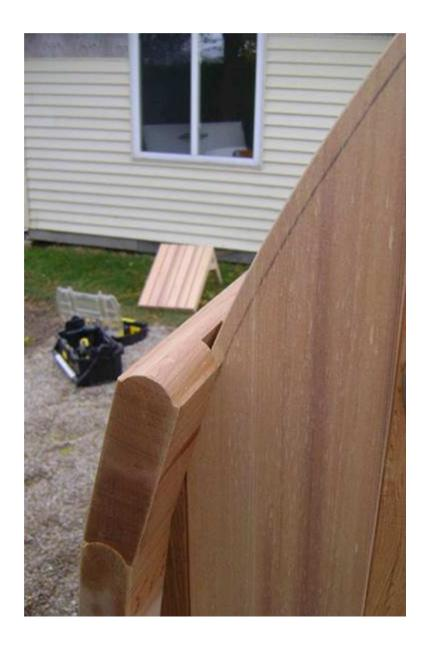
Again, make sure the inside faces of the staves line up with the pencil circle on the end walls. Once you get them to hold onto the edge of the wall, by themselves or with nails, tap them in or out with a hammer to line them up with the pencil line.
