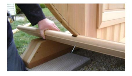
Here the installer is using one of the supplied 2½" finishing nails to hold a stave onto the bottom part of the barrel. You may not need to use nails, as sometimes the staves stay on without nails.
