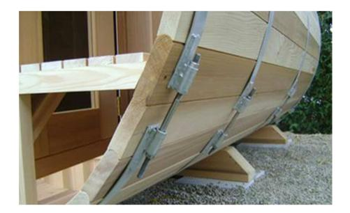
Rotate the bands so that the tightening hardware is at the desired location. Usually this is the least visible area of the barrel. That could be bottom centre if you don't mind crawling down under to tighten them.
