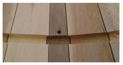
A half-inch hole was bored for drainage just inside the walls on the lower special stave.
