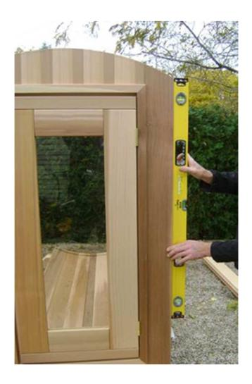
Get the middle front and back wall segments plum using a carpenter's level, or a plumb bob.
