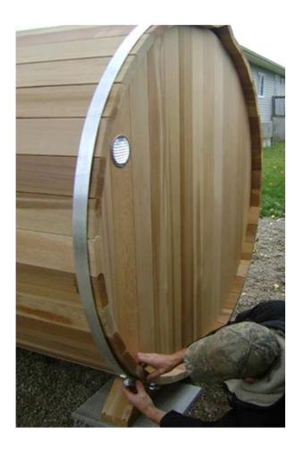
Here the band is being placed with the tightening hardware on the bottom of the side that is least visible.
