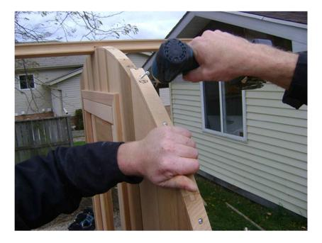
Fasten the half-moon side wall segments to the middle wall segments with supplied 2½" screws.
