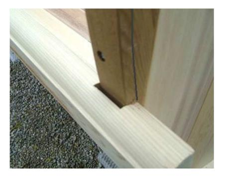
Once the front and back end walls are assembled, start to assemble the barrel.
