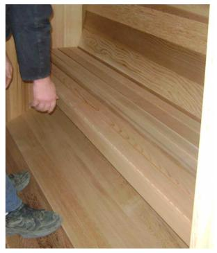
Fasten the inside benches atop the pre-installed brackets on the walls (2½" screws).
