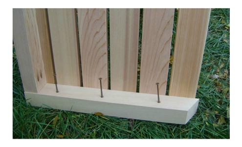
Start the long screws (2½") into the end brackets to make installation easier...
