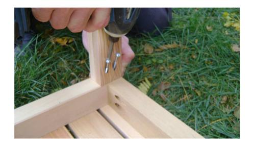
Assemble the outside benches for saunas with the porch option using supplied 1½" screws into and predrilled holes.
