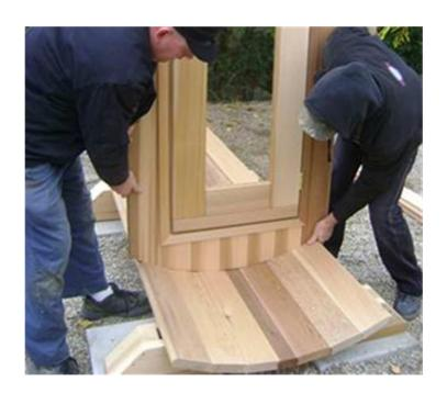
Place the middle sections of the end walls into the groove in the staves.
