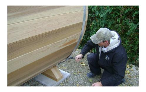
Now tighten the bands, each a little at a time. If you have two people assembling, one should tighten while the other bangs down on the bands, (or up from inside the chamber if necessary) to keep the circular shape.
