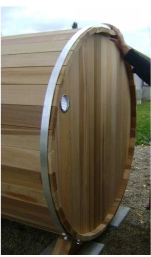
Finish installing the staves on the top half.
