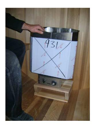
The heater goes on the centre of the end wall, close to the floor. Place something under the heater to position it with the bottom of the heater close to the floor, and mark the bracket positions on the wall. The heater will hang on the brackets when installed.
