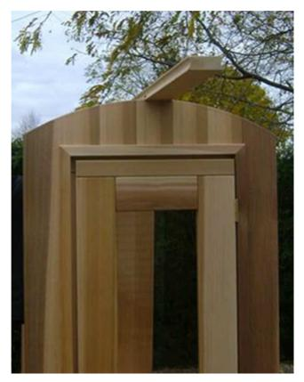
Put the special top stave in place to help stabilize the wall sections.
