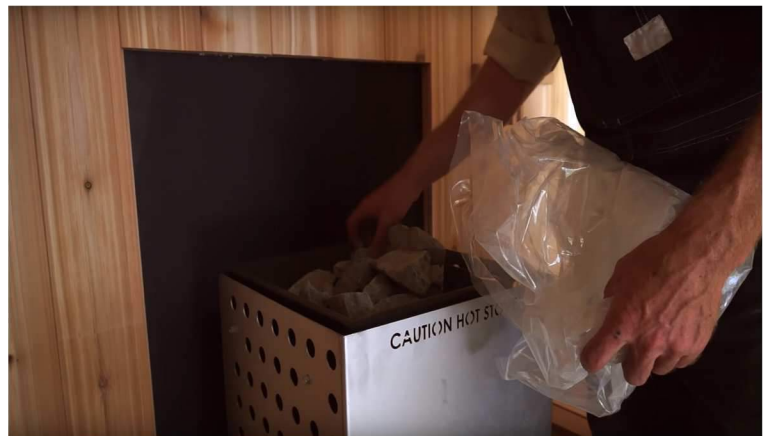
WB-6. Space rocks out evenly in top of heater. * Operate the heater for an hour with the sauna door fully open to burn off any residual coating from the manufacturing process before using.
