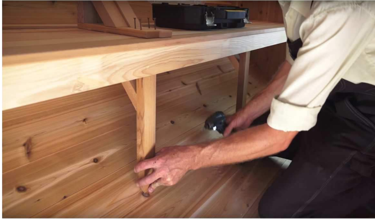
33. Space out the bench supports evenly under the bench.
