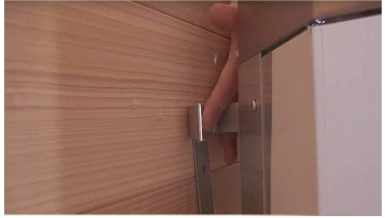
EH-2. Mark the placement of the heater brackets.
