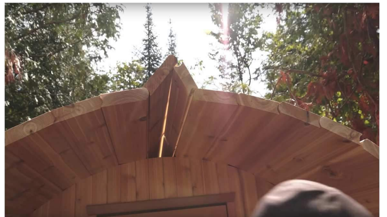
20. When you reach the top, you will find that the last wall stave doesn't look like it fits properly. This is normal.
