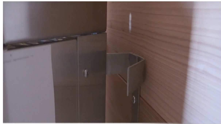
EH-4. Place heater on wall brackets.
