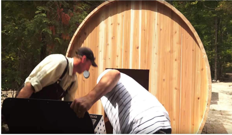
WB-1. To install the wood burning heater, get help to lift heater into the hole in the back of the sauna.
