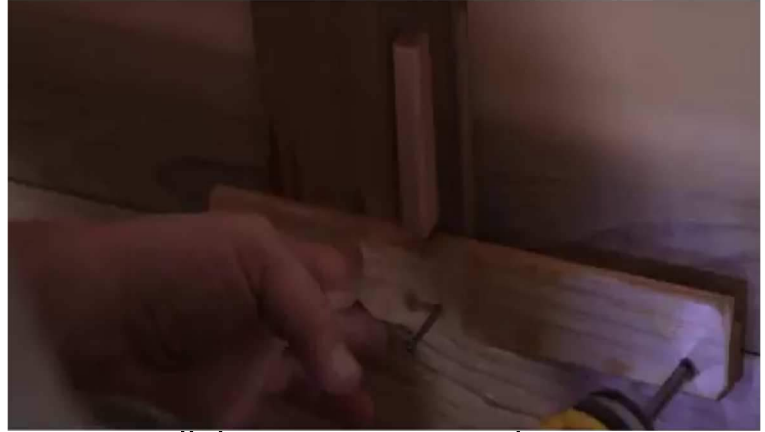
46. To install the vent cover, use the cover as a guide, level the lower rail and fasten with 1 1/2" screws.
