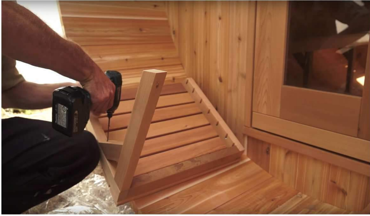
39. To install the porch seats, screw the legs into the end of the seats with 2 1/2" screws. Attach brace with 2 1/2" screw.
