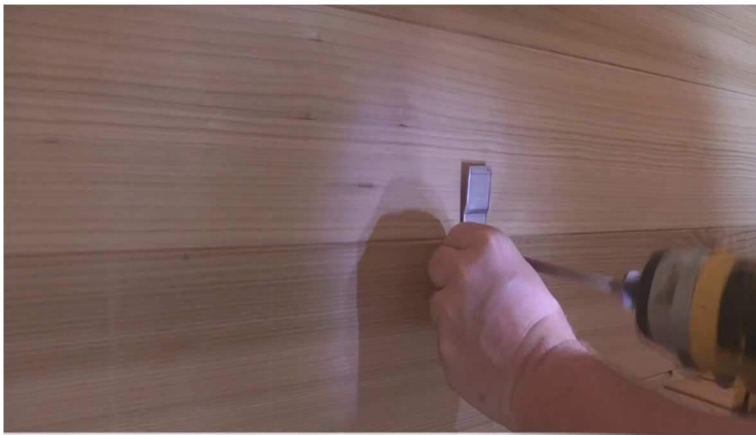
EH-3. Attach heater brackets to back wall of sauna using 1 1/2" screws.
