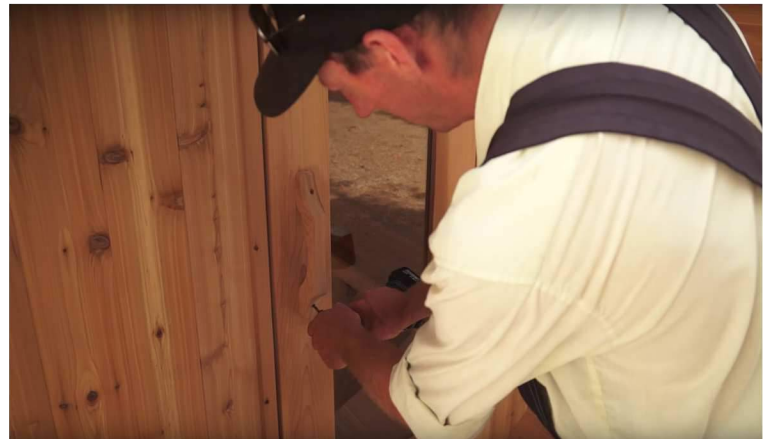
36. Center outer door handle on outside of door and secure with 2" screws. *Magnets are very strong and may require some force to pull door open for first time.
