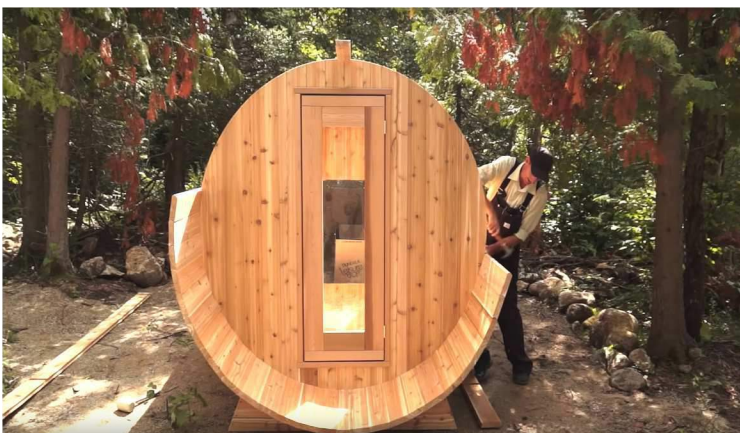
19. Continue to add staves on both sides to the top.
