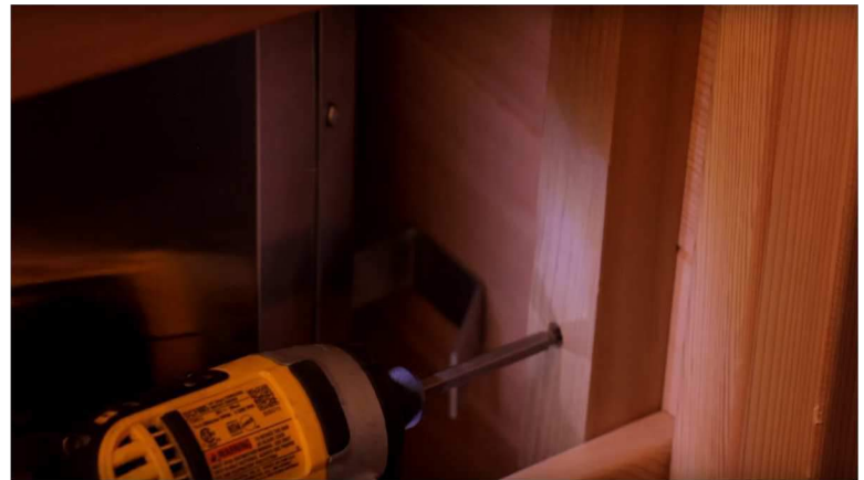
HG-4. Using 2 1/2" screws in pre drilled holes, fasten guard to back wall.
