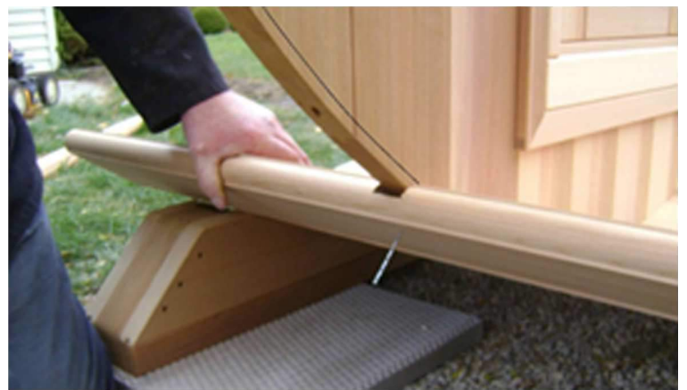
18. When installing staves, tap tightly together while leaving as much of a gap as possible between stave and wall as in picture. This will make the tightening of the bands easier.
