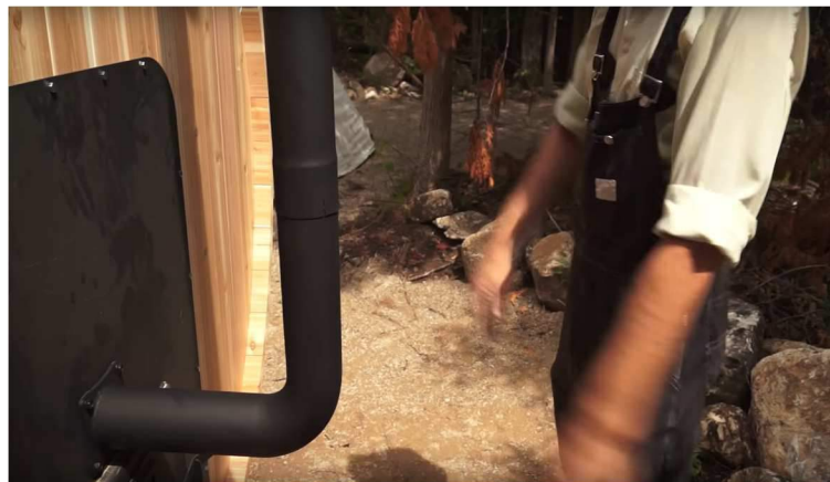
WB-5. Insert the flanged end of the chimney head onto the elbow firmly. * Some finessing may be required. * Wash the rocks thoroughly before placing them into the heater.
