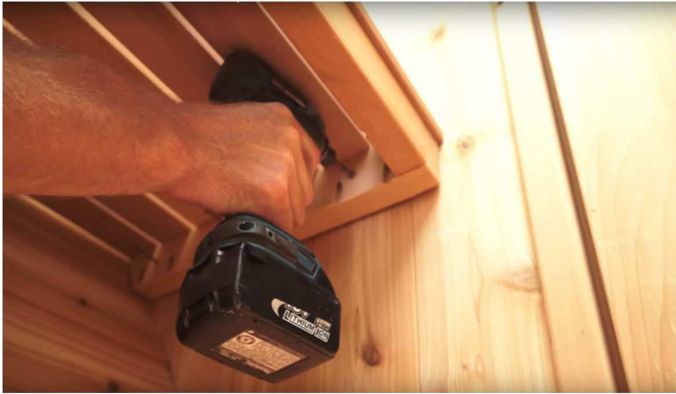
41. Secure the porch seat to wall with 2 1/2" screws.
