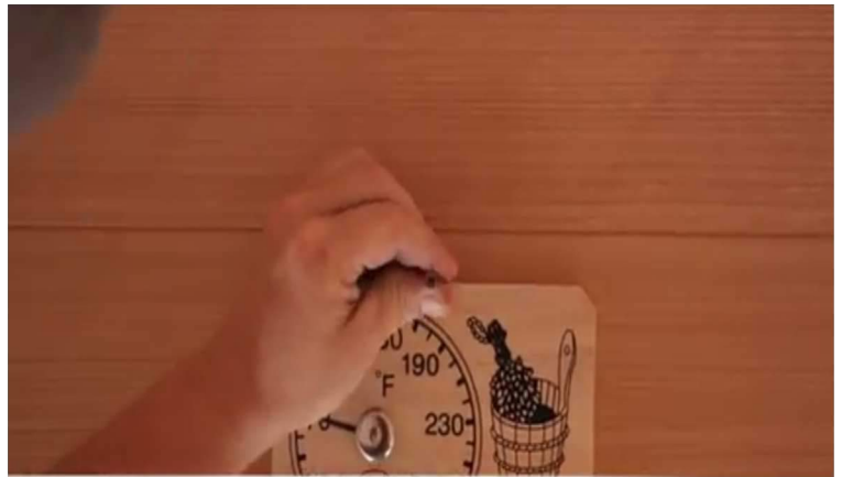
48. Install the thermometer centered above the door using a 1 1/2" screw.
