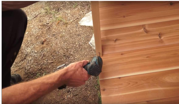
43. Secure leg to floor with 2 1/2" screw as well.
