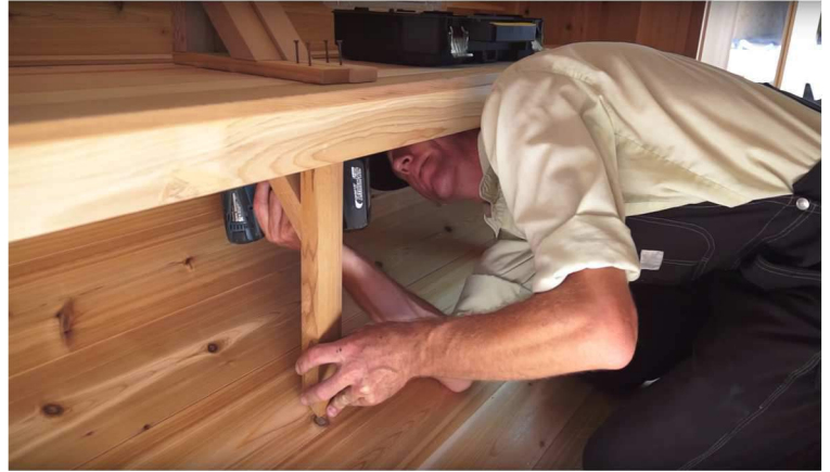
34. Secure the support to the bench using 1 1/2" screws from underneath.
