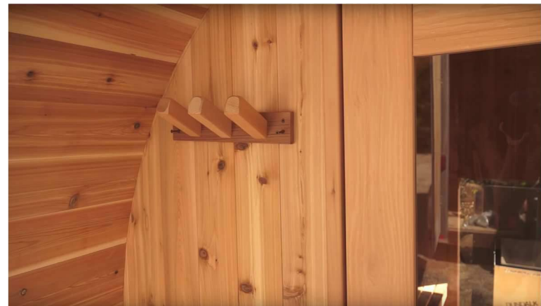
38. Install towel hanger at desired height on outer wall using 1 1/2" screws.
