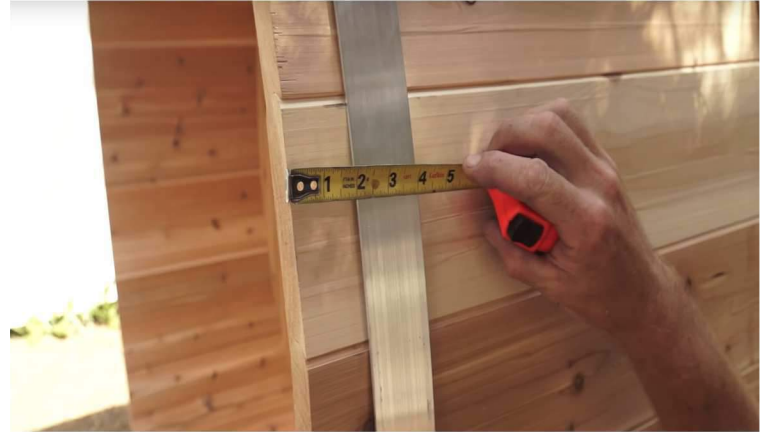
28. The front and back bands should be 2" from the stave ends. * Space out middle bands according to sauna size and how many bands are included.
