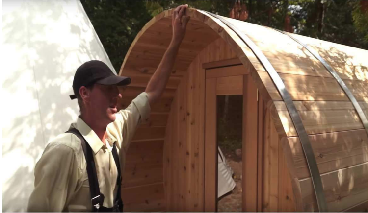
27. Make sure ends of sauna are flush.
