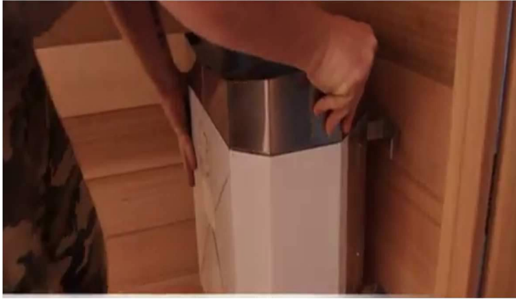
EH-1. Place heater on top of the included box of sauna rocks to get the correct height for installation.
