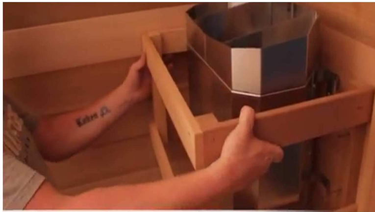
HG-3. Place heater guard around electric heater. *Make sure heater guard is level before securing.
