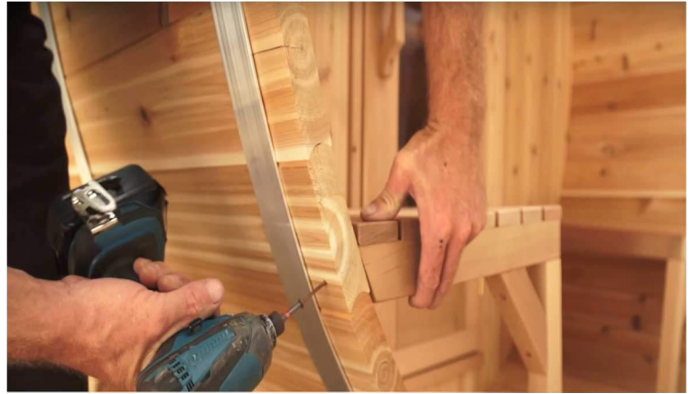
42. On outer side of porch seat, secure seat from outside of sauna with 2 1/2" screw.
