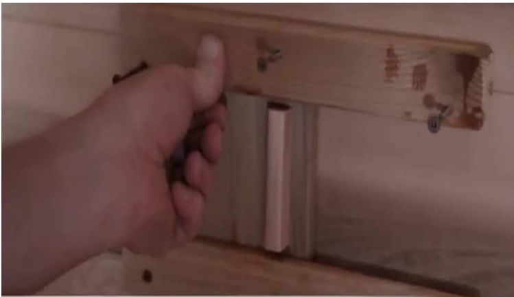
47. Make sure when securing the top vent cover rail that the vent cover can still move with ease. *Be careful not to overtighten.
