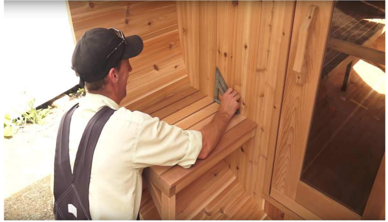
40. Use a square or level to make sure porch seat is level.
