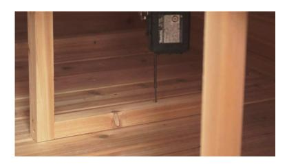
Secure the bottom of each bench support to the floor using 2½" deck screws, front and back.
