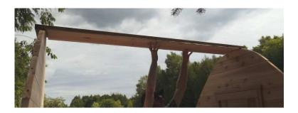
Centre the top piece on top of the walls and fasten it using two 1½" deck screws on each end.
