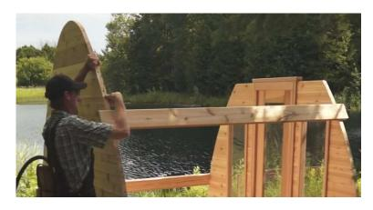
Centre the top section of the back wall and fasten at the bottom corners with  $2\frac{1}{2}$ " deck screws.
