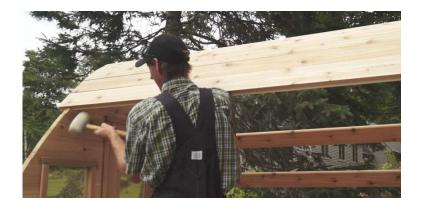
**Install the wall boards from the top down**, tapping them into place with a rubber mallet.
