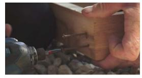
Align the floor joists with the X's on the floor frame, so that the sides of the joists line up with the lines beside the X's. Fasten with two 3" wood screws on each end.
