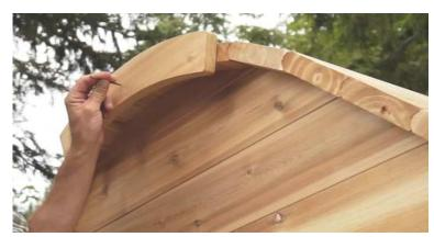
Install the front and back trim boards as shown using supplied 1%" deck screws. Place the screws approximately every third wall board.
