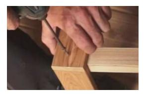
Assemble the cedar heater guard fence using 2½" deck screws.
