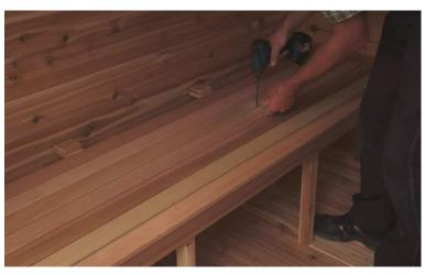
Place 2½" deck screws between the bench boards, front and back, at each support.
