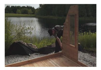
Locate and position the **back bottom wall assembly** (picture left) flush with the back edge of the floor.
