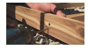
Now it is time to fasten the floor boards. Start by laying a floor board groove-side into the notch in the front side of the floor frame. Continue laying down the boards and tap them tight together with a mallet. Don't worry if there is a gap left over at the back wall when the last board is put in place as that will be covered by the back wall. Drive one 1 ½" deck screw at each intersection with the floor joists.
