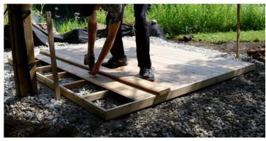
Preparing the base. Crushed limestone gravel: Clear loose vegetation and soil, level the ground, lay down weed barrier cloth if desired, and fill the area with 2-4" of <u>crushed</u> limestone gravel. Level and tamp. Patio stones on top are an option but not necessary.
