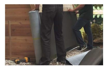
Roll out the underlay (Ice and Water Dam Shield) and cut each length about one inch longer than the length of the wall boards.
