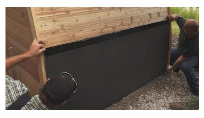
Place a piece as shown, with the **black front side adhesive strip** oriented towards the top. Peel and fold back the top 3 or 4 inches of the backing from the top edge, and stick in place so that the bottom edge is flush with the bottom of the sauna wall.
