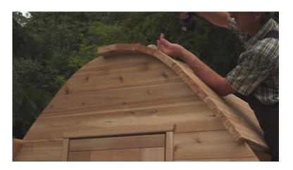
Secure the wall boards in place using 2½" deck screws where they join the front and rear walls.
