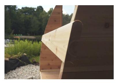
Use a wall board as a brace to steady the wall segments, as shown, to hold the wall segments in place until the roof is in place.
