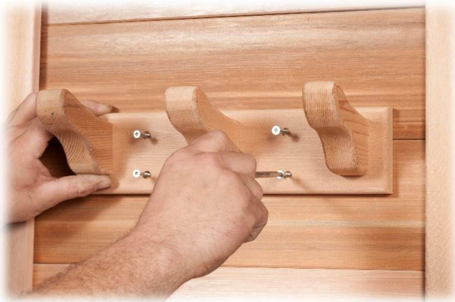
Fig. 7.1 Four #2 Robertson flathead wood screws
